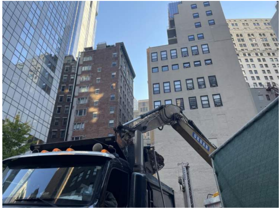
Photo 1: View of Urban loading a tri-axial truck with soil/fill for off-site disposal (facing east).
