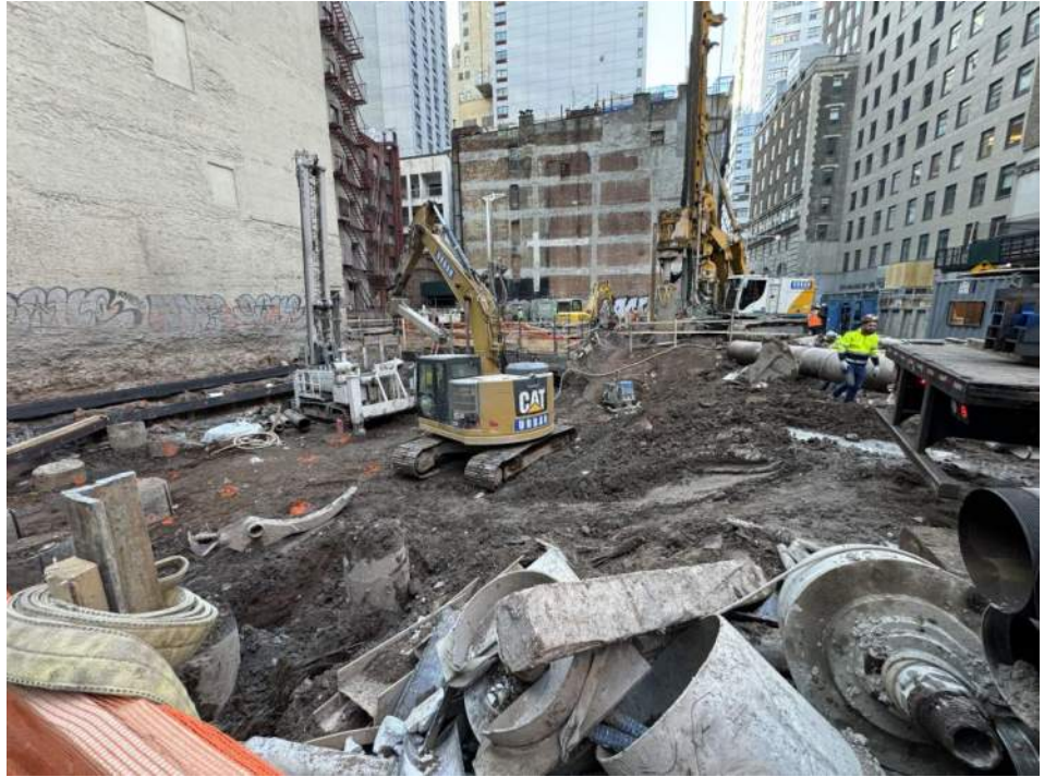
Photo 1: General view of the site (facing south).
