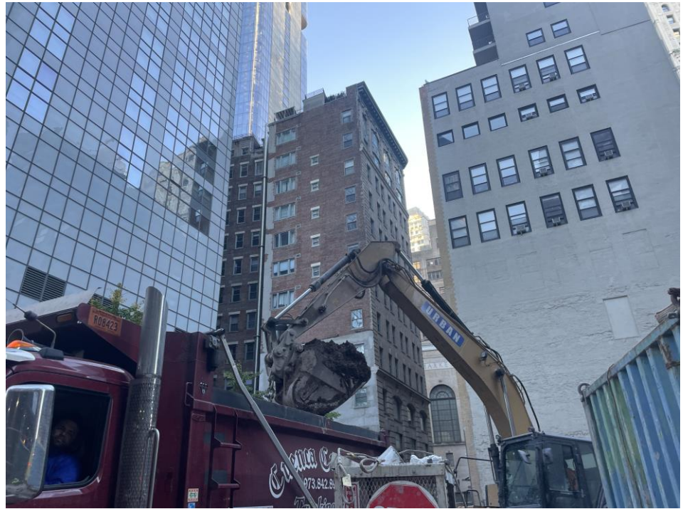
Photo 1: View of Urban loading tri-axial truck for off-site disposal in the northwestern part of the site (facing northeast).
