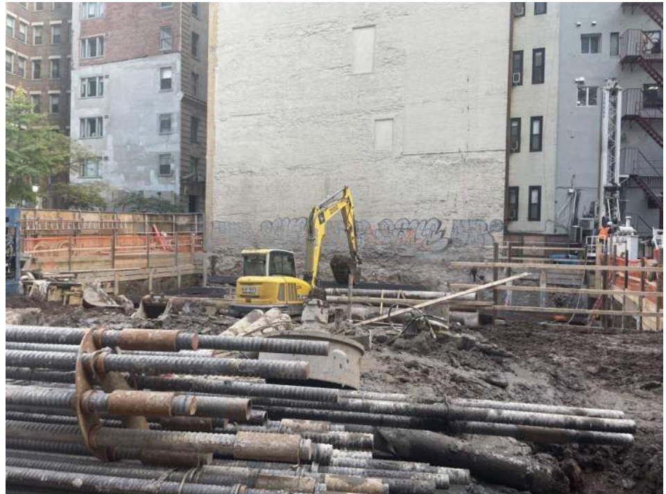
Photo 2: View of Urban excavating soil/fill in WC03_5-10 (facing east).
