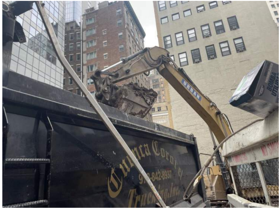
Photo 1: View of Urban loading tri-axial truck with soil/fill for off-site disposal (facing northeast).
