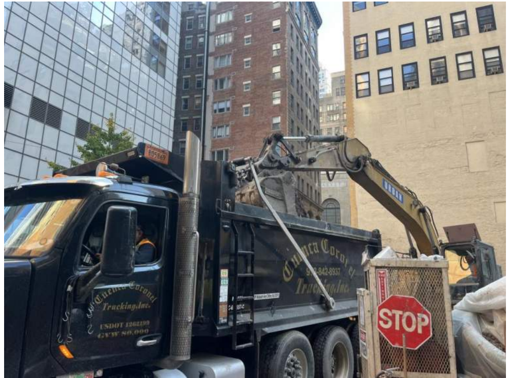
Photo 1: View of Urban loading tri-axial truck for off-site disposal in the northwestern part of the site (facing northeast).
