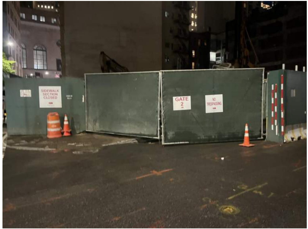
Photo 3: View of the site entrance/exit at the corner of Carlisle and Washington Street at the end of the work day (facing southeast).
