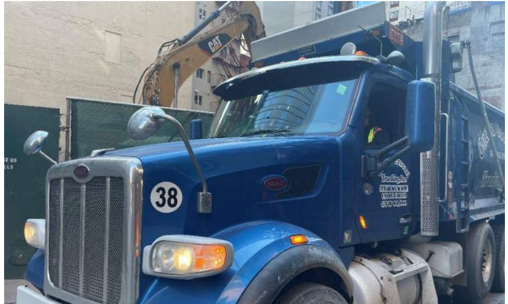
Photo 1: View of Urban loading soil/fill for off-site disposal (facing southeast).
