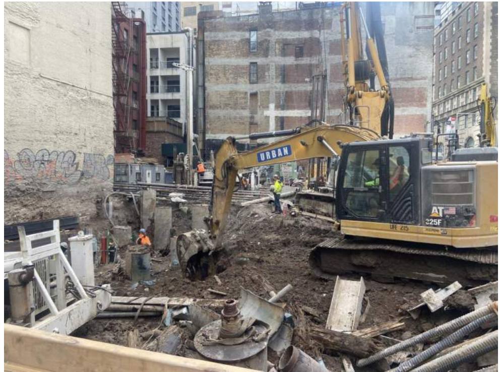
Photo 1: View of Urban excavating soil/fill in grid WC03 (facing southeast).
