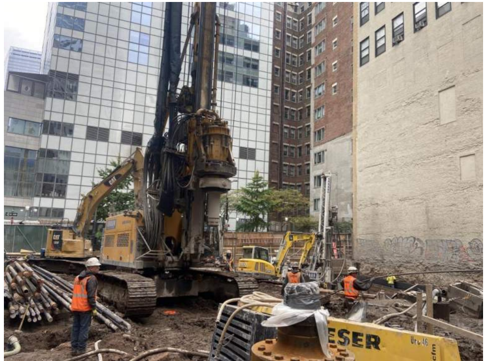
Photo 2: General view of the site (facing northeast).
