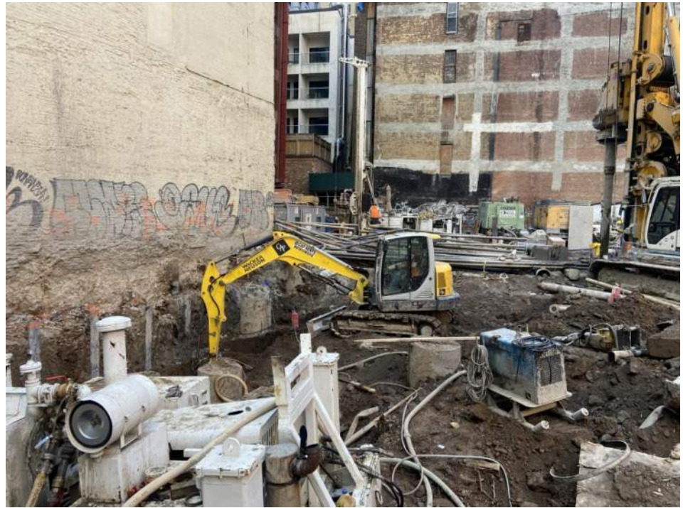
Photo 1: View of Urban excavating soil/fill in WC03_5-10 (facing south).
