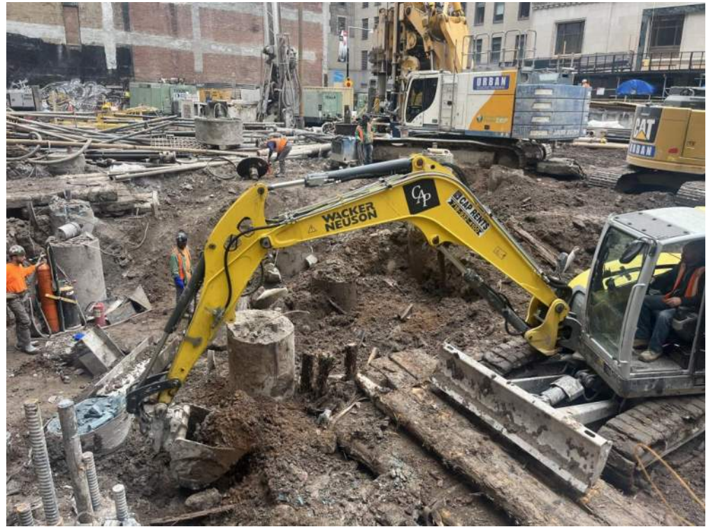
Photo 1: View of Urban excavating soil/fill in WC03_5-10 (facing northeast).
