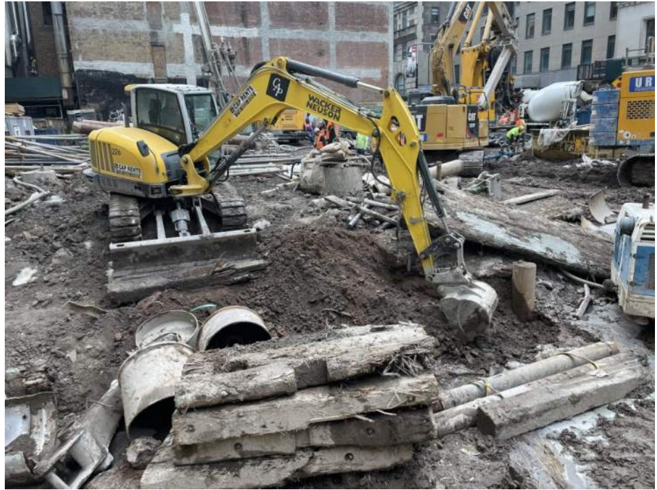
Photo 1: View of Urban excavating soil/fill in WC03 (facing south).
