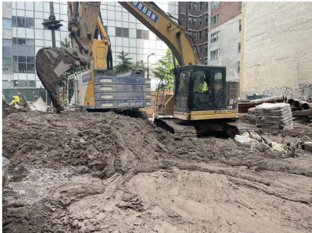
Photo 2: View of the Urban stockpiling excavated soil/fill in WC03 (facing northeast).
