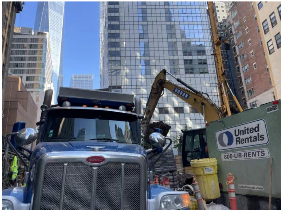
Photo 2: View of Urban loading a truck with soil/fill for off-site disposal (facing north).
