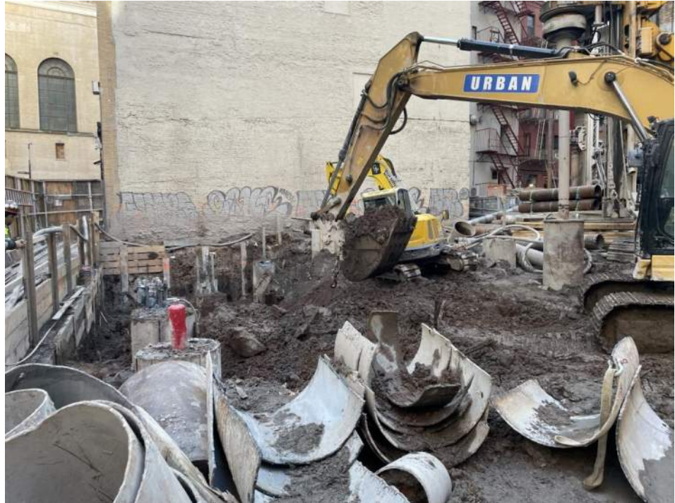
Photo 1: View of Urban excavating soil/fill in WC03 (facing east).
