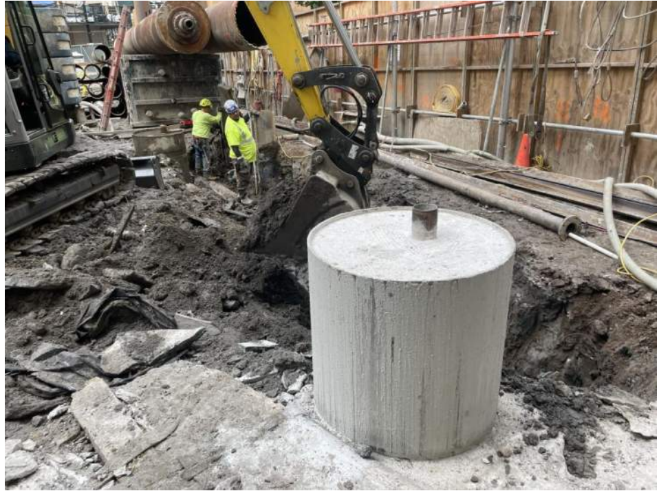
Photo 1: View of Urban excavating soil/fill in WC03 (facing northwest).
