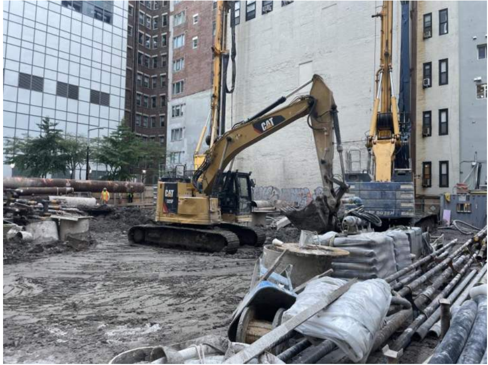
Photo 1: General view of the site (facing northeast).
