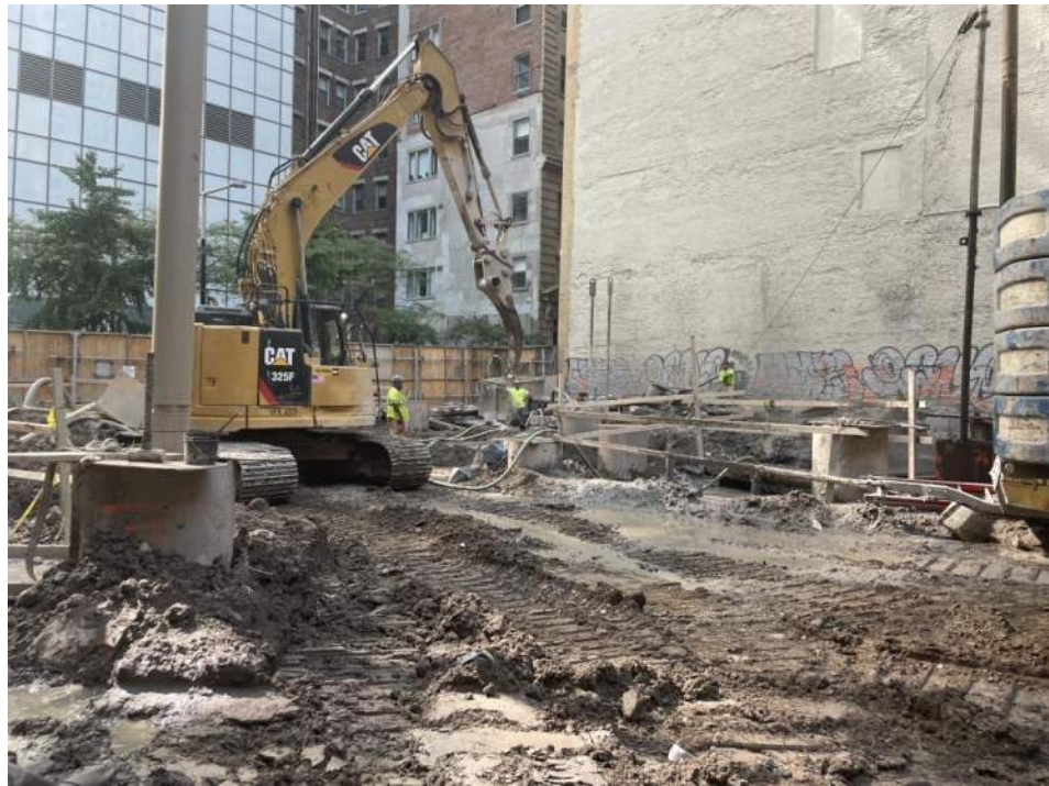
Photo 2: View of Urban excavating soil/fill in waste characterization grid WC03 (facing northeast).
