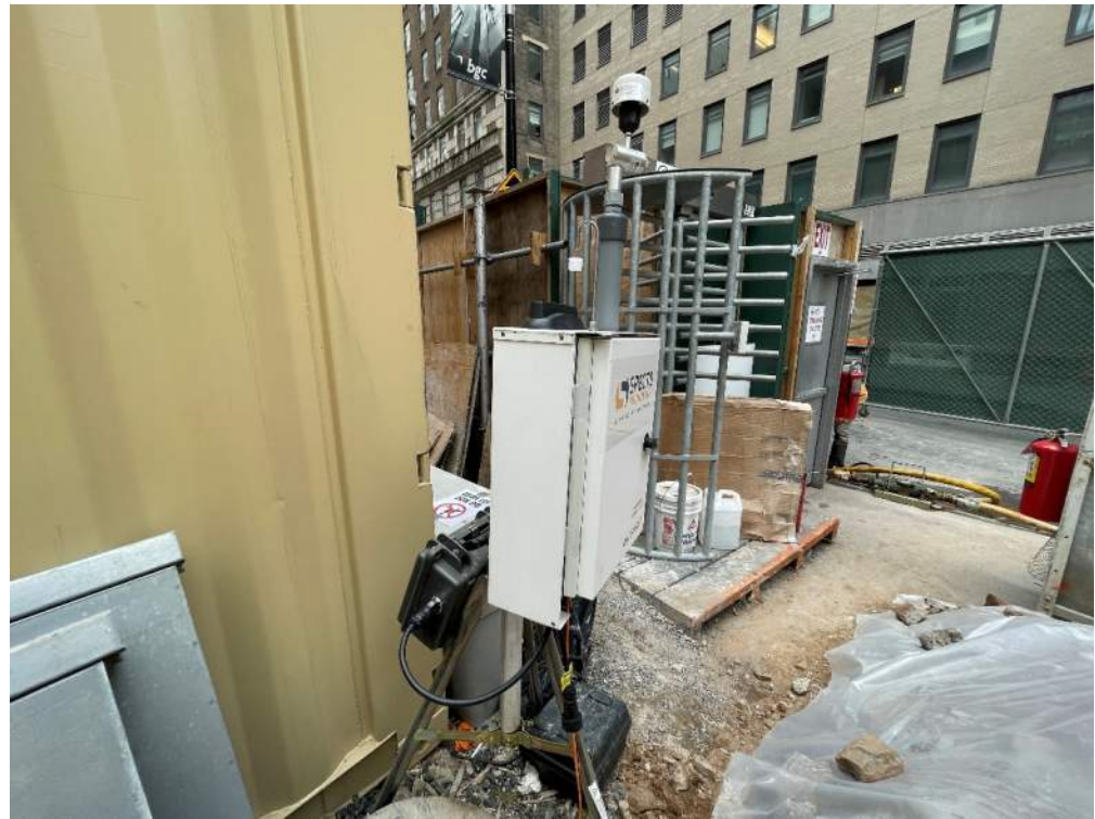
Photo 3: View of CAMP Station 2 in the southwestern part of the site (facing southwest).
