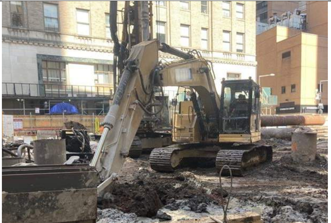
Photo 2: Urban excavating soil/fill in waste characterization grid WC03 (facing northwest).
