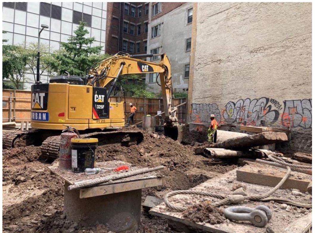
Photo 2: Urban excavating soil/fill in waste characterization grid WC03 (facing northeast).
