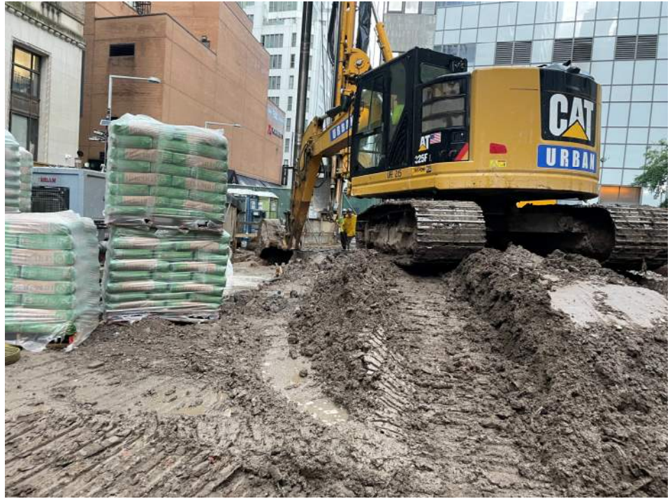
Photo 1: Urban excavating soil/fill in the western part of WC02 (facing north).
