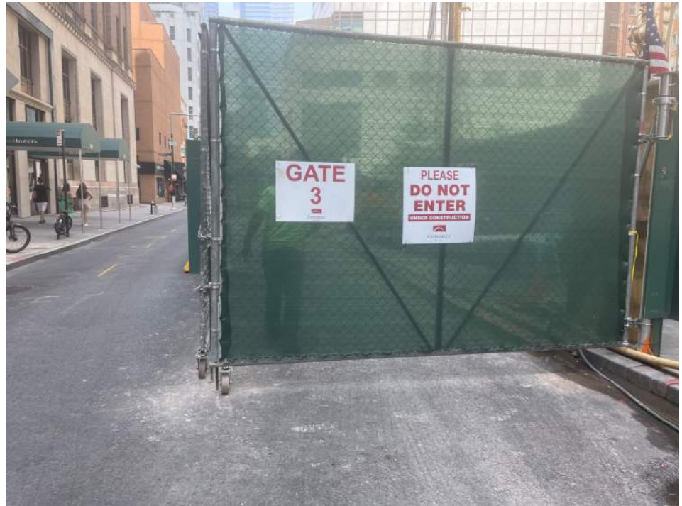
Photo 5: View of the entrance/exit of the site along Washington Street at the end of the work day (facing northeast).
