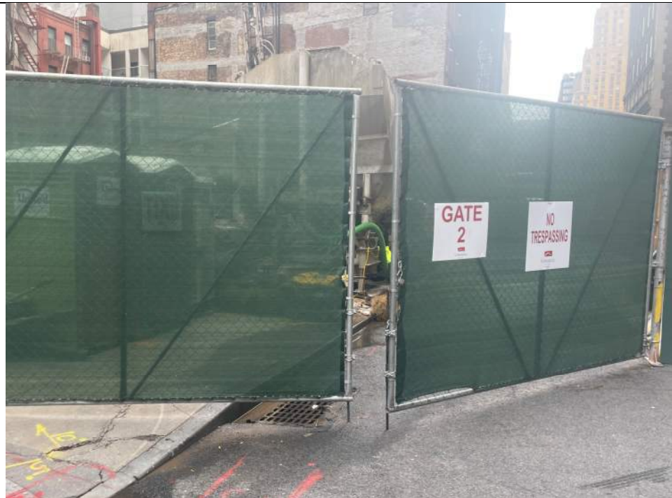
Photo 6: View of the entrance/exit of the site at the corner of Carlisle and Washington Street at the end of the work day (facing south).
