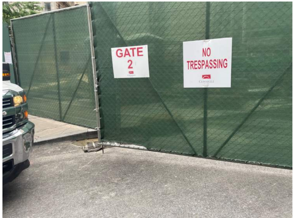
Photo 8: View of the entrance/exit of the site at the corner of Carlisle and Washington Street at the end of the work day (facing southeast).
