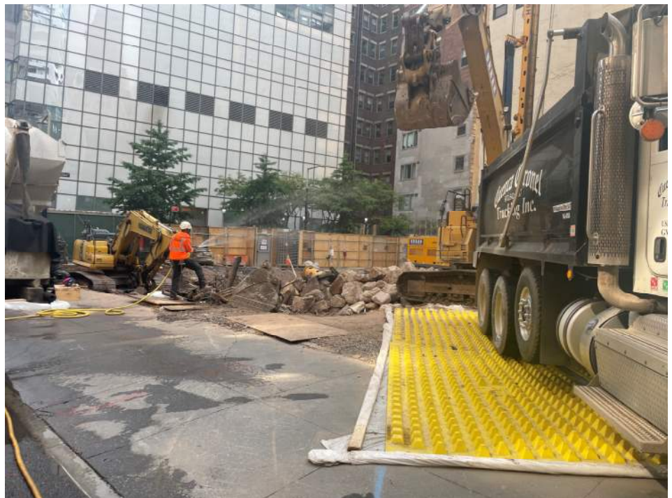
Photo 2: Urban spraying water for dust suppression while loading C&D debris for off-site disposal in the southern part of WC02 (facing northeast).
