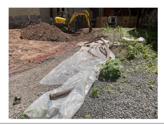
**Photo 4:** Overhead view of the concrete encasement of the UST encountered within the excavation area in WC04 and WC05.
