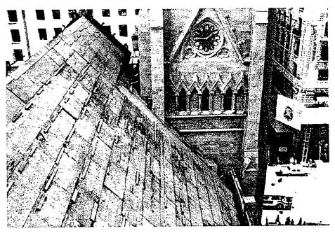
Figure 4. Dropped equipment, tools, and materials all present risks when new construction rises above neighboring historic structures. In this case, the historic state roof was completely covered with sheets of exterior grade plywood. Photo: National Park Service files.
