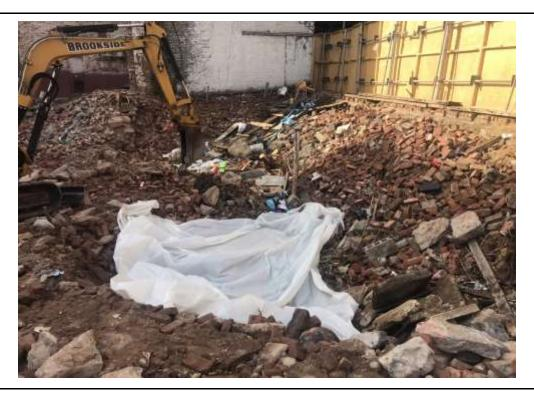
Photo 15: Placement of polysheeting over AST staging area and stained soil as a demarcation layer for future remediation, facing west. 15 March 2022.
