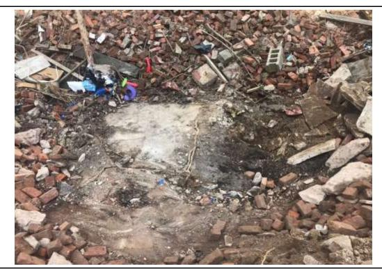
Photo 13: Concrete pad removal with stained soil and secondary clean concrete pad below AST staging area, facing northeast. 15 March 2022.
