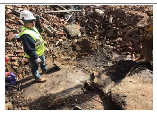
Photo 12: Concrete pad removal with stained soil and secondary clean concrete pad below AST staging area, facing northeast. 15 March 2022.
