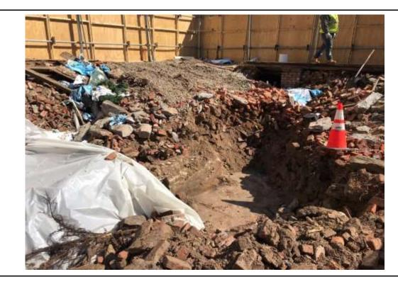
Photo 6: Concrete slab below original AST location, facing southeast. 14 March 2022.
