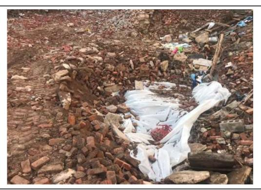
Photo 16: Placement of polysheeting over AST staging area and stained soil as a demarcation layer for future remediation, facing west. 15 March 2022.
