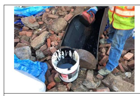
Photo 2: Removal of remaining tank sludge, facing west. 14 March 2022.
