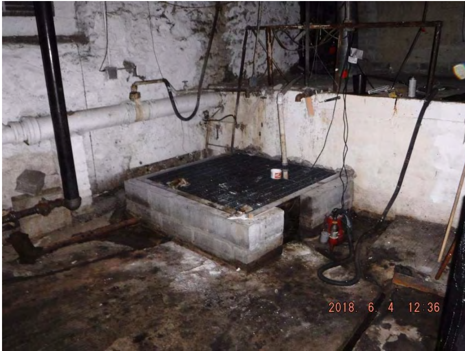
Photograph 1: Sump pit in the basement boiler room.
