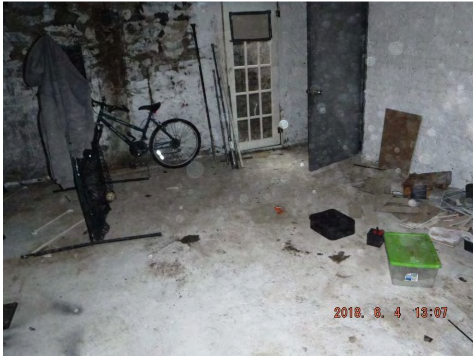
Photograph 1: Location of B1 at the south end of the former dry cleaner space (patched area in floor)
