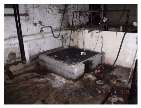
**Photograph 1:** Sump pit in the basement boiler room.
