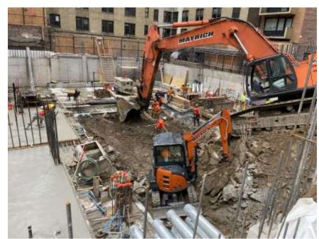
Photo 2: View of Mayrich removing chipped bedrock from the central part of the site (facing southwest).
