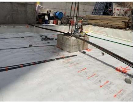
Photo 1: View of Mayrich installing waterproofing in the southwestern part of the site (facing west).
