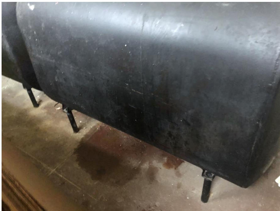
Photo 2: View of stained concrete beneath the leaking AST in the Lot 60 cellar (facing east).
