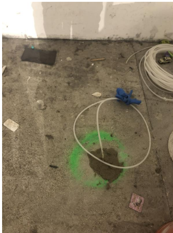
Photo 2: Installed sub-slab vapor point (SSV08) located in Lot 59 (facing west).
