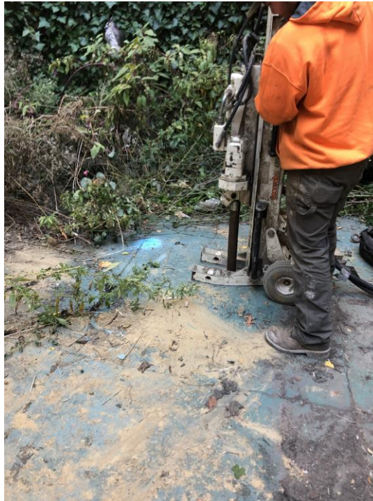
Photo 1: View of AARCO installing SV07 in Lot 60 (facing southwest).
