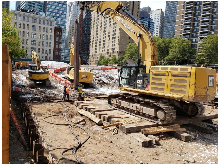
Photo 1: CCJV installing a steel sheet pile for SOE system installation in the southeastern part of the site (facing northwest)
