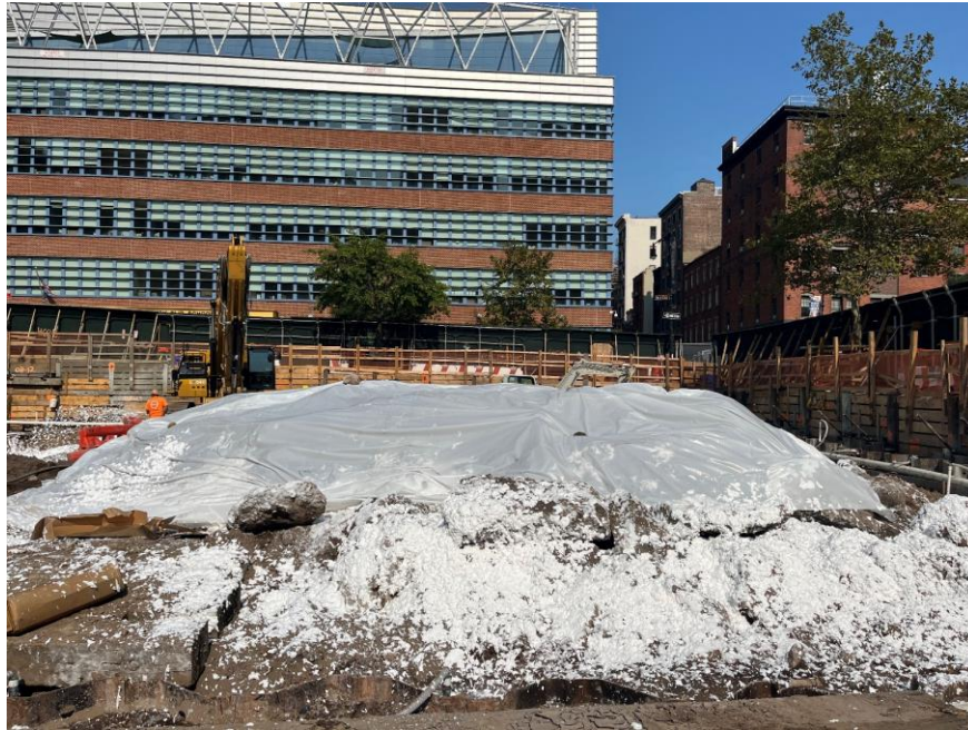
Photo 1: Petroleum-impacted soil/fill stockpile covered in Atmos® AC-645 dust/vapor suppressing foam and polyethylene sheeting in the southeastern part of the site (facing east)
