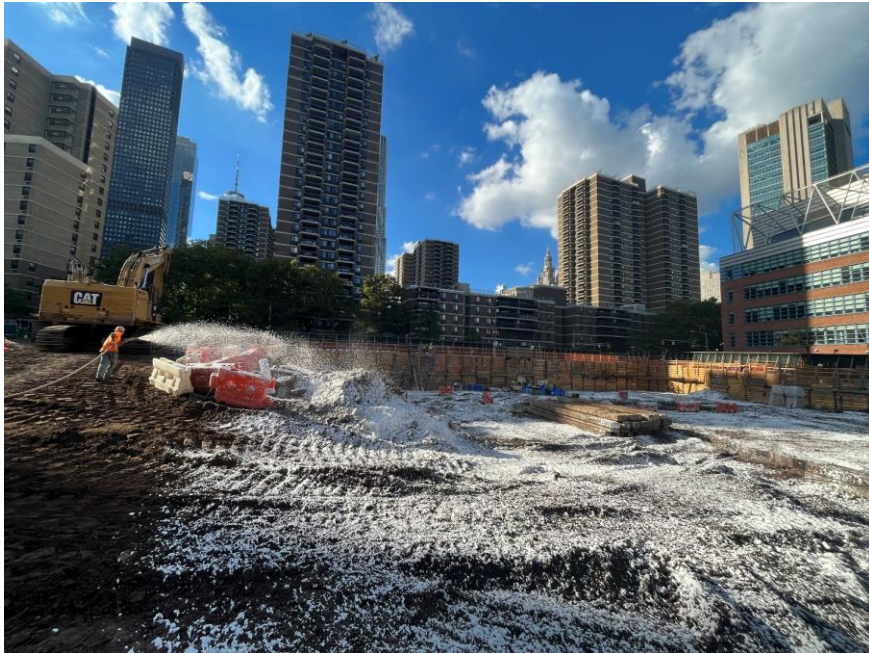
Photo 2: CCJV applying Atmos® AC-645 dust/vapor suppressing foam to exposed soil/fill to create a temporary overnight cover (facing north)
