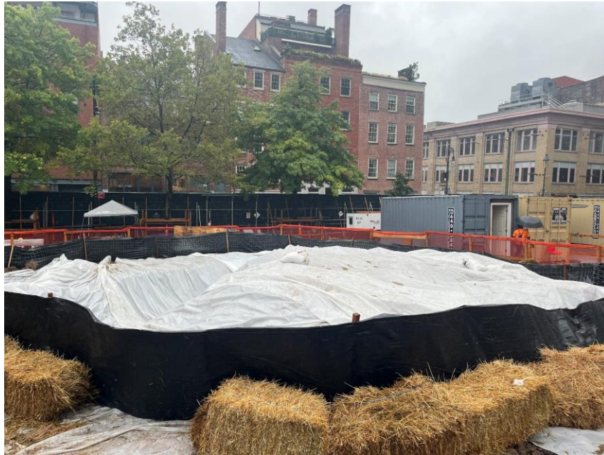
Photo 1: Hazardous lead-impacted soil/fill stockpile covered with polyethylene sheeting and surrounded with silt fencing and hay bales in the southwestern part of the site (facing southwest)
