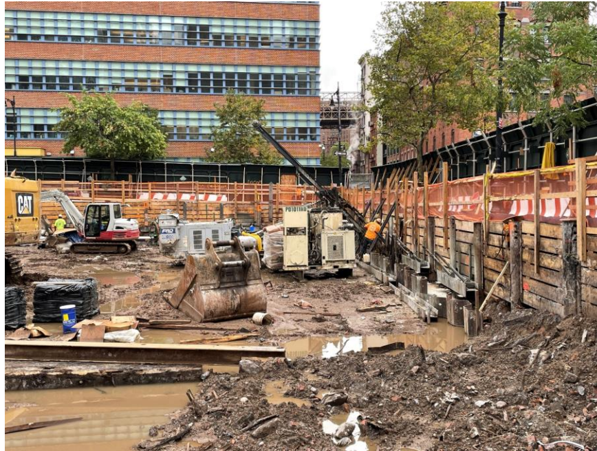
Photo 1: CCJV installing a tie-back along the southern boundary of the site (facing southeast)
