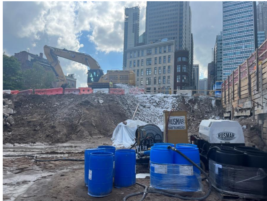
Photo 2: CCJV applying Atmos® AC-645 dust/vapor suppressing foam to exposed soil/fill in the northern part of the site (facing west)
