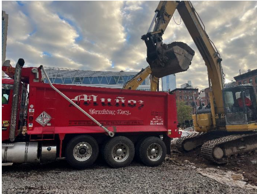
Photo 1: CCJV loading hazardous lead-impacted soil/fill into a tri-axle truck for off-site disposal (facing east)
