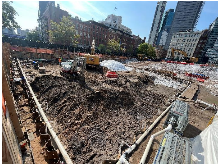
Photo 2: CCJV excavating petroleum-impacted soil/fill in the southeastern part of the site (facing southwest)
