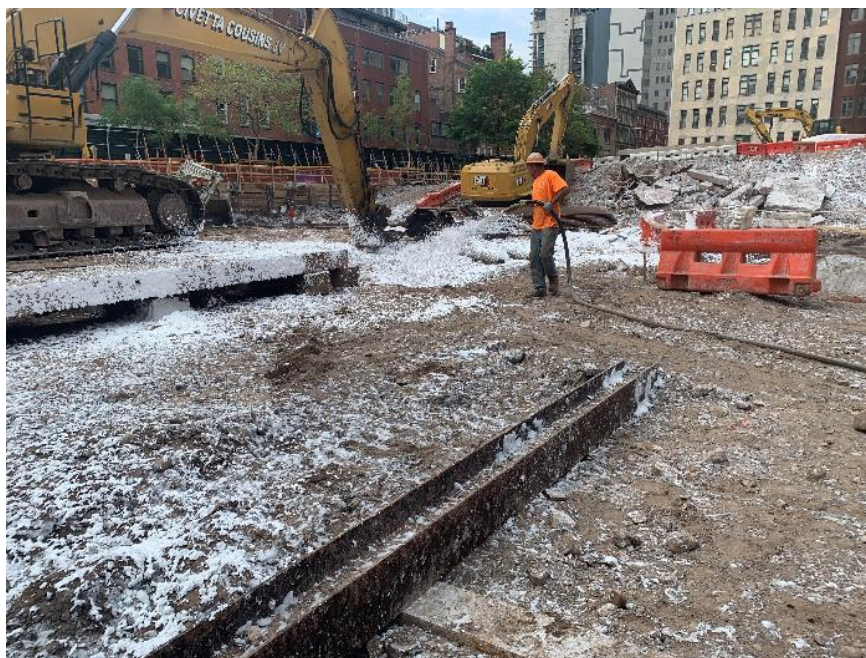
Photo 1: CCJV applying Atmos® AC-645 dust/vapor suppressing foam to exposed soil/fill across the site (facing southwest).
