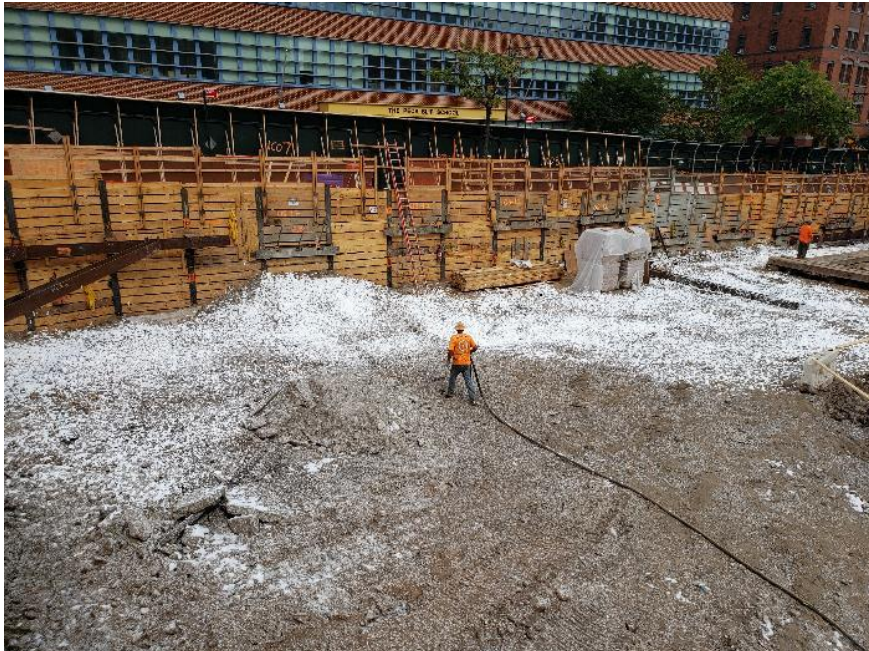
Photo 2: CCJV applying Atmos® AC-645 dust/vapor suppressing foam to exposed soil/fill in the eastern part of the site (facing southeast).
