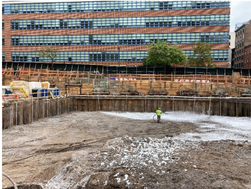
Photo 1: CCJV applying Atmos® AC-645 dust/vapor suppressing foam for reinstallation of the temporary overnight cover (facing east).
