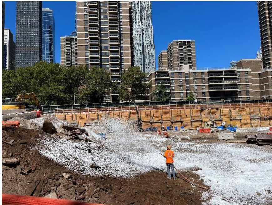
Photo 2: CCJV applying Atmos® AC-645 dust/vapor suppressing foam to exposed soil/fill during excavation in the south-central part of the site (facing north).
