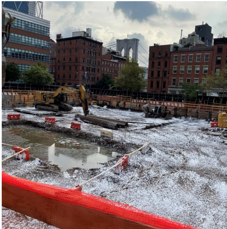
Photo 1: Atmos® AC-645 dust/vapor suppressing foam applied to exposed soil/fill across the site (facing southeast)
