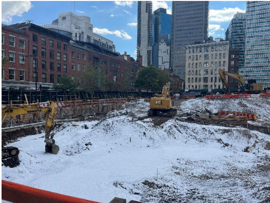
Photo 2: Atmos® AC-645 dust/vapor suppressing foam applied to exposed soil/fill for the temporary overnight cover (facing southwest)
