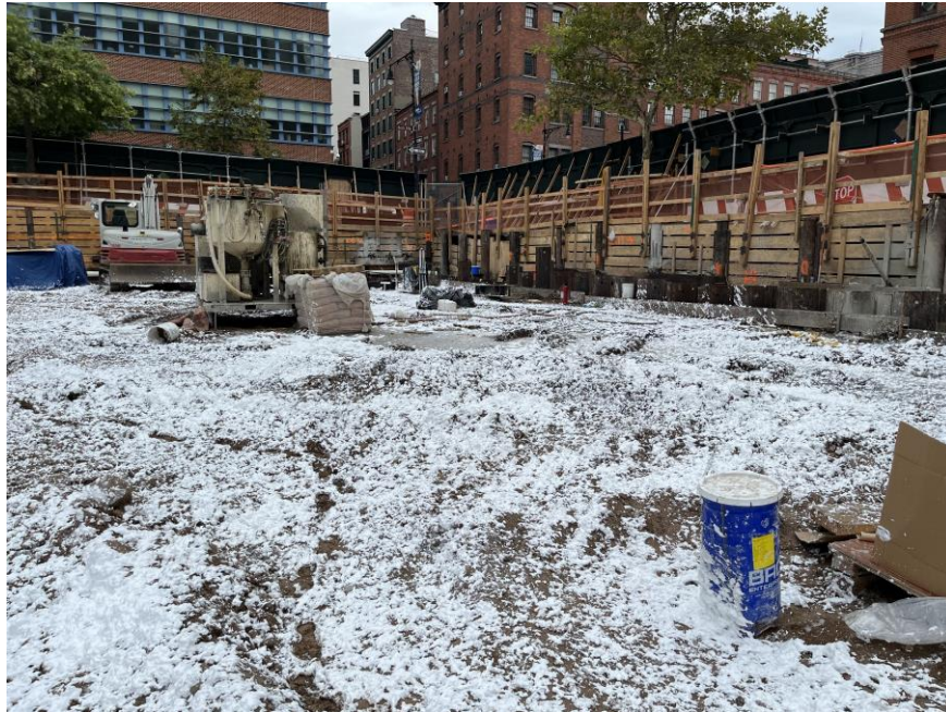
Photo 1: Atmos® AC-645 dust/vapor suppressing foam applied to exposed soil/fill in the southeastern part of the site (facing southeast)
