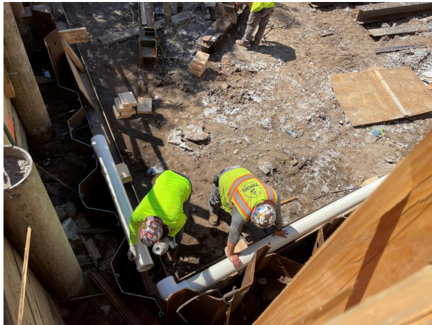
Photo 2: Tristate Groundwater installing the dewatering system in the southeastern part of the site (facing northwest)
