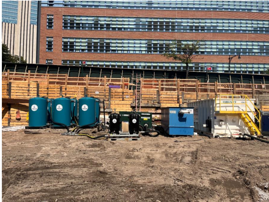
Photo 1: Dewatering system components in the eastern part of the site (facing east)
