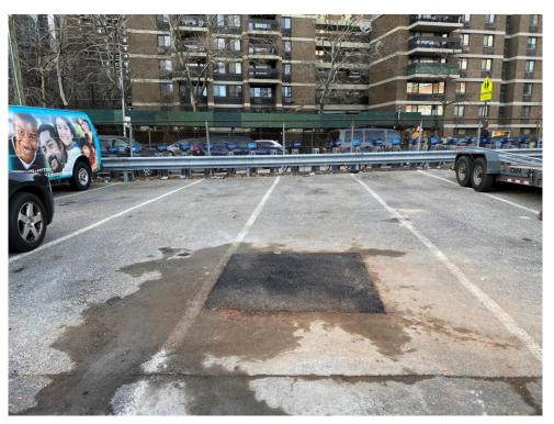
Photo 15: View of test pit TP05, restored to match the surrounding grade surface using cold patch asphalt (facing north) (02/12/2022)
