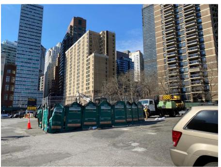
Photo 2: View of typical work zone fencing with chain-link fence and Echo Barrier H9<sup>™</sup> acoustic curtains (facing northwest).
