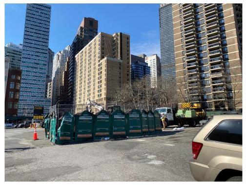
Photo 2: Work zone fencing with chain-link fence and Echo Barrier H9<sup>™</sup> acoustic curtains (facing northwest) (02/12/2022)
