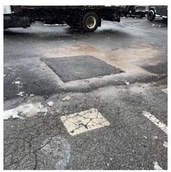
Photo 4: View of test pit TP04, restored to the surrounding grade using cold patch asphalt (facing north).
