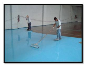
Application of Retro-Coat SEALANT to a 20 mil total thickness
