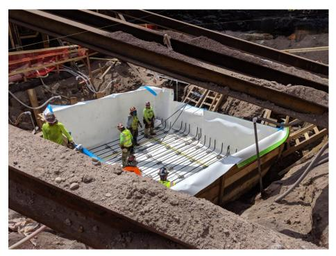
Photo 40: View of Men of Steel installing rebar in Grid 4, facing southeast (7/11/2019)
