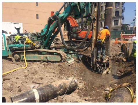
Photo 12: View of Moncon drilling soldier pile S24, facing north (8/7/2018)
