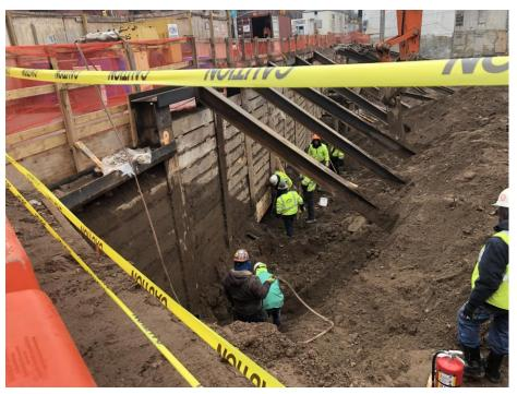
Photo 22: View of Moncon installing lagging along eastern site boundary in Grid 2, facing southeast (2/18/2019)
