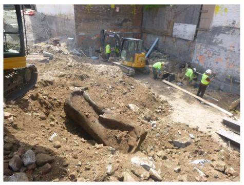
Photo 8: View of 550-gallon steel UST uncovered in Grid 1 during excavation activities, facing south (6/20/2018)
