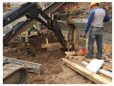
Photo 13: View of Moncon excavating in Grid 4 (7-13) for underpinning installation, facing east (8/17/2018)
