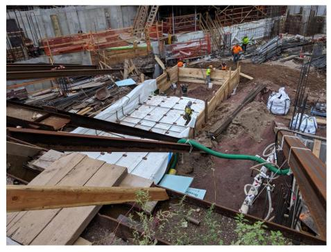
Photo 42: View of DripDrop installing Grace Preprufe® 160R Plus and 300R Plus waterproofing membrane in Grid 4, facing southwest (8/19/2019)
