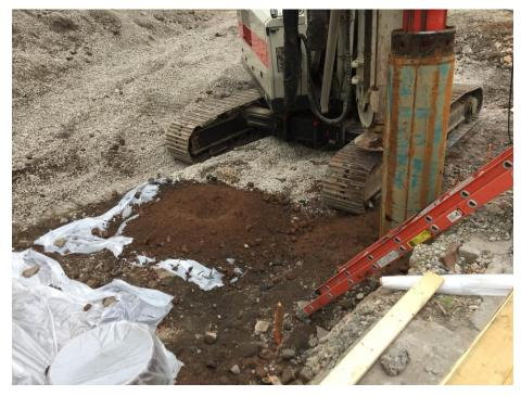
Photo 4: Moncon installing soldier pile S7 casing, facing northwest (5/31/2018)
