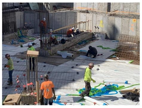
Photo 48: View of DripDrop installing Grace Preprufe® 300R Plus waterproofing membrane in Grid 3, facing southwest (9/29/2019)
