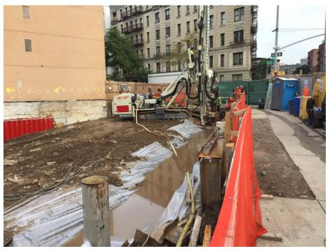
Photo 16: View of Moncon drilling production pile 22 in Grid 3, facing north (10/4/2018)
