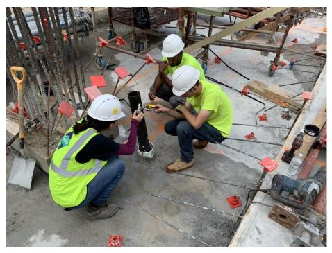
Photo 50: View of Hydrotech installing a sampling port in the riser pipe, facing southeast (10/02/2019)
