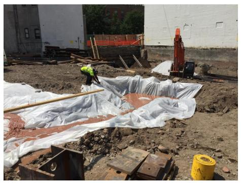
Photo 14: View of polyethylene-lined trench and retention pond, facing southwest (8/24/2018)
