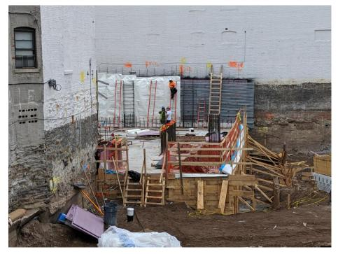
Photo 27: View of DripDrop installing Grace Preprufe® 160R waterproofing membrane on western wall of Grid 3, facing west (5/17/2019)
