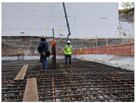
Photo 26: View of Rise pouring concrete for 36-inch reinforced slab in the southern portion of Grid 3, facing west (5/14/2019)
