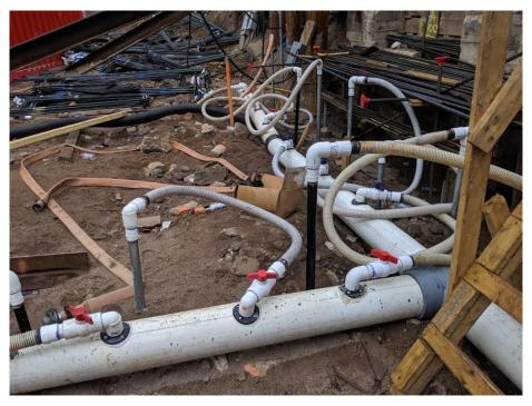
Photo 36: View of dewatering system in Grid 2, facing north (7/5/2019)
