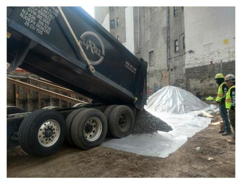
Photo 24: View of Rise importing ¾-inch virgin stone from RockTech of New Jersey, facing southeast (4/11/2019)
