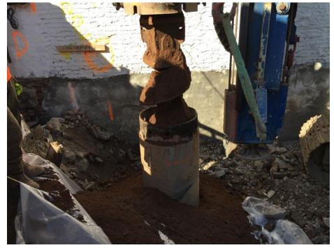
Photo 9: View of Moncon drilling soldier pile S0 in Grid 4, facing south (6/25/2018)
