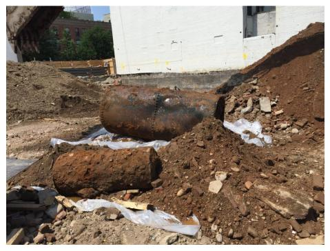
Photo 10: View of a 50-gallon and a 550-gallon steel USTs uncovered during excavation and staged on polyethylene sheeting, facing west (7/11/2018)
