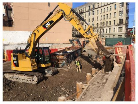
Photo 18: Moncon backfilling behind timber lagging with approved reuse material from Grid 3 (17-20), facing northwest (11/8/2018)
