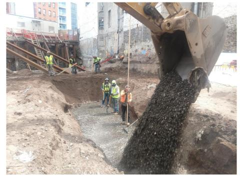
Photo 25: View of Rise backfilling excavation with <sup>3</sup>/<sub>4</sub>-inch virgin stone in Grids 3 and 4 between 19 and 20 feet bgs, facing southeast (4/30/2019)
