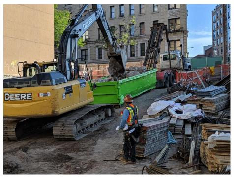
Photo 28: View of Rise loading concrete into dumpster for off-site disposal, facing northwest (5/22/2019)
