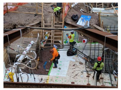
Photo 41: View of DripDrop installing Grace Preprufe® 300R Plus in Grid 4, facing west (8/6/2019)
