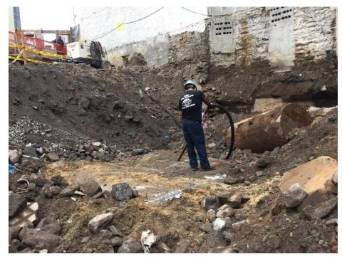
Photo 17: View of ABC Tank Repair and Lining, Inc. (ABC) pumping contents of UST11, facing southwest (10/9/2018)
