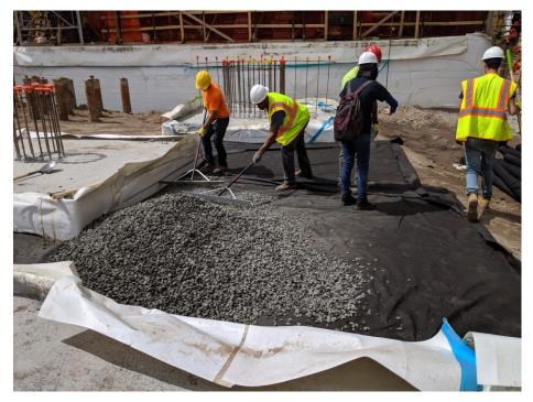
Photo 31: View of Hydrotech spreading ¾-inch virgin stone from Tilcon – West Nyack Quarry on geotextile fabric for SMD system installation in Grid 3, facing south (6/7/2019)
