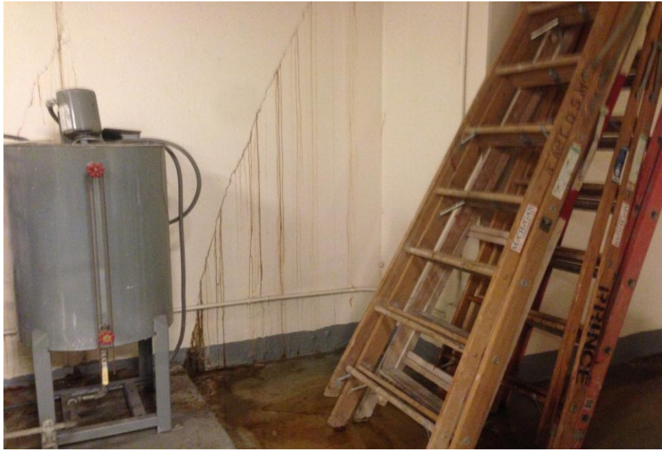
Photo 1: Walls of River Place II sub-cellar showing observed intrusion
