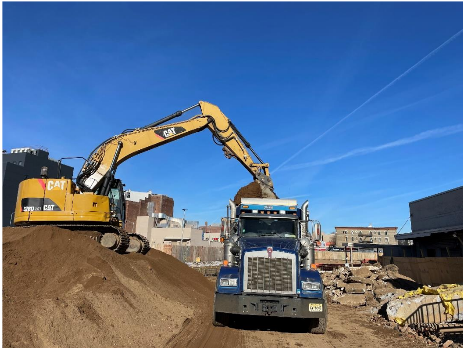
Photo 2: View of contractor loading soil in Lot 14, facing north.
