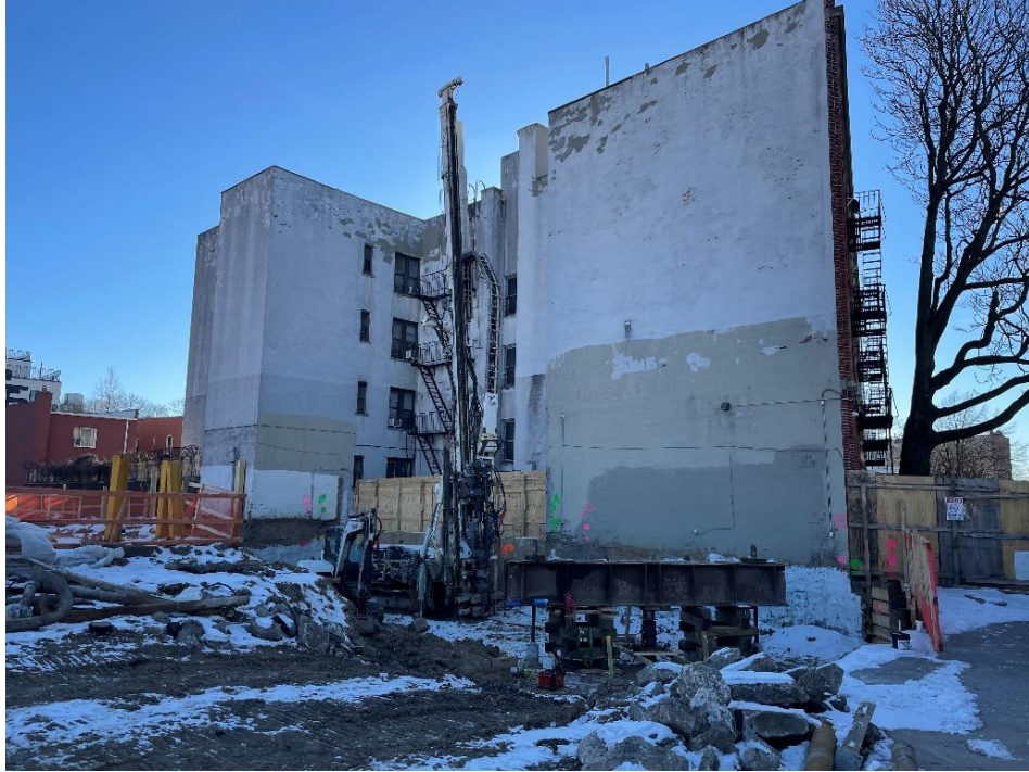
Photo 1: View of piles installation on Lot 53, facing south-southeast.
