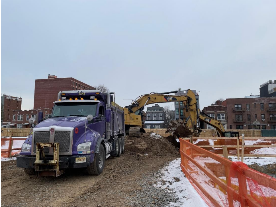
Photo 1: View of soil disposal in Lot 53, facing east.
