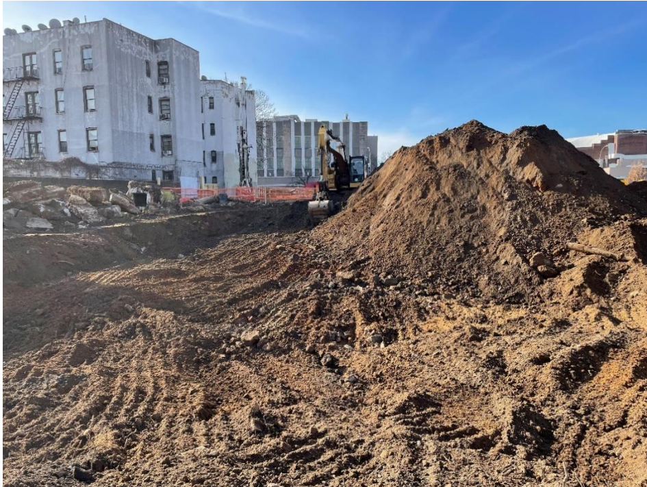
Photo 2: View of soil stockpile in Lot 53, facing south.
