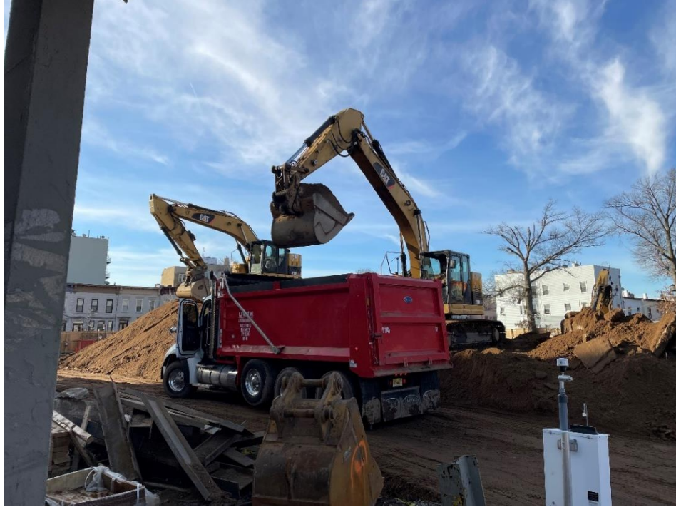
Photo 1: View of soil disposal in Lot 14, facing southwest
