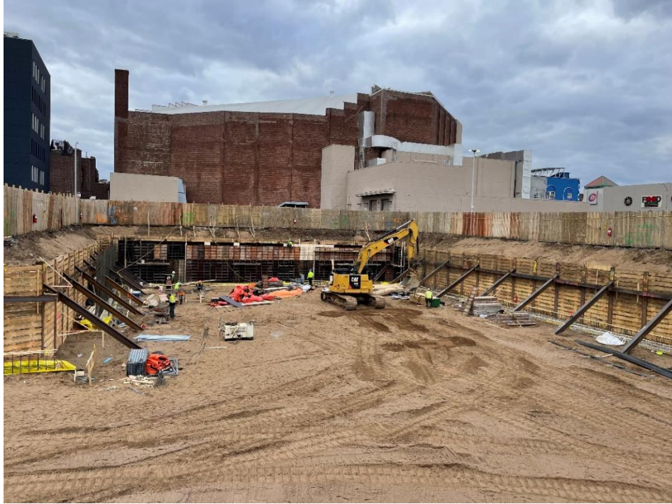
Photo 1: View of SOE activities in Lot 14, facing west.
