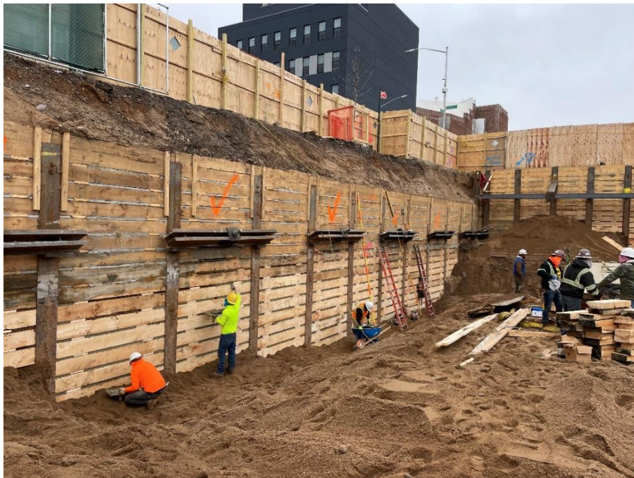
Photo 2: View of SOE activities in Lot 14, facing southwest.
