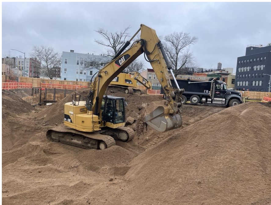
Photo 2: View of the contractor grading Site soils in Lot 14, facing west.
