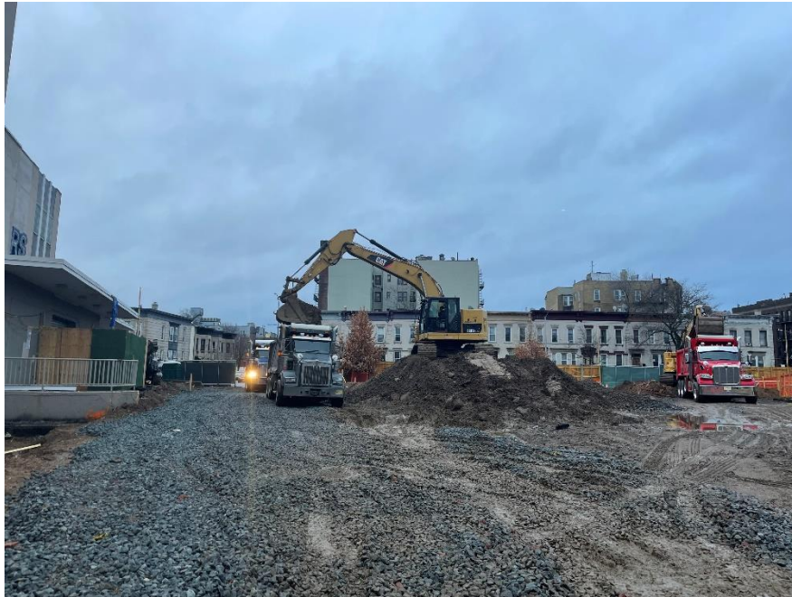
Photo 1: View of soil loadout on Lot 14, facing south-southwest.
