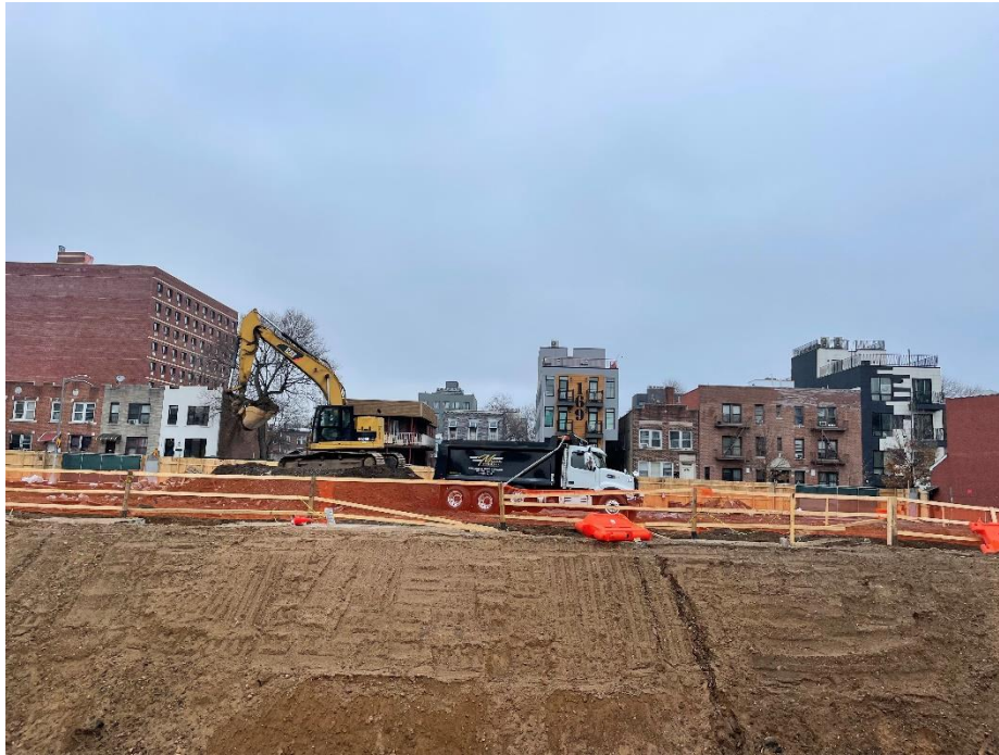
Photo 1: View of contractor loading asphalt in Lot 53, facing east.
