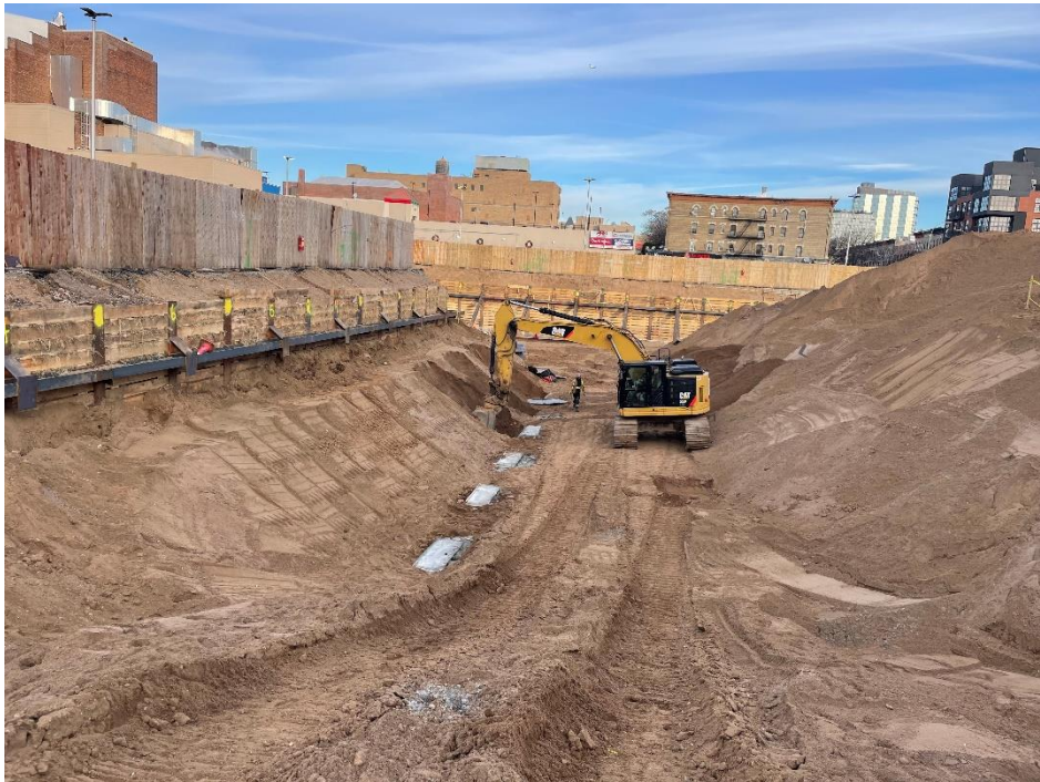
Photo 2: View of SOE activities in Lot 14, facing north.
