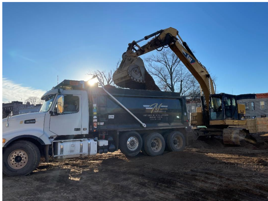
Photo 2: View of contractor loading soil on Lot 14, facing west-southwest.
