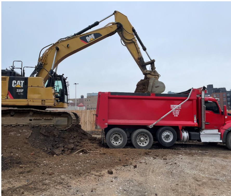
Photo 2: View of contractor loading soil from Lot 14, facing northwest.
