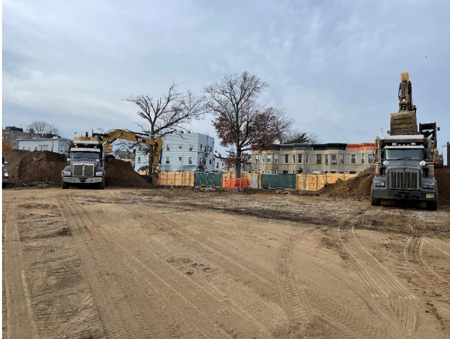
Photo 1: View of contractor loading soil from Lot 14, facing southwest.
