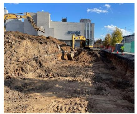
Photo 2: View of excavation for SOE installation along the southern perimeter of lot 14, facing east.
