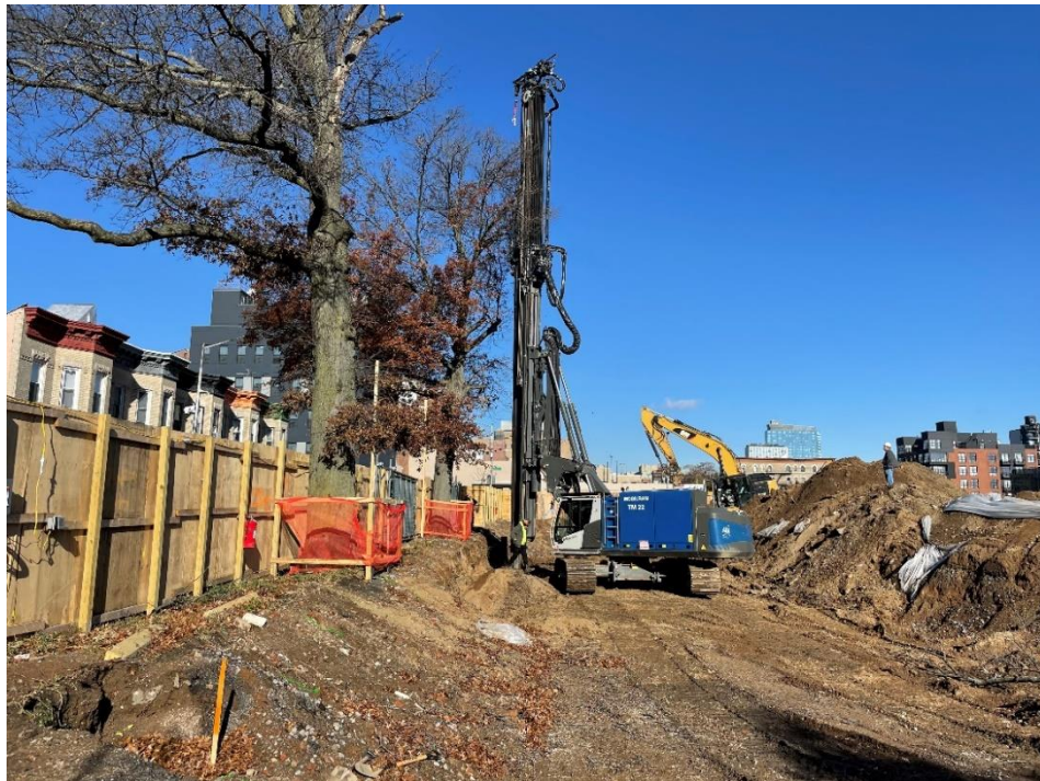
Photo 2: View of contractor installing H piles in Lot 14, facing north.
