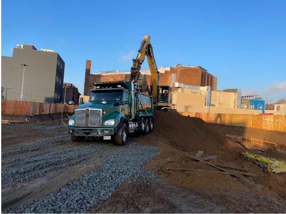
Photo 1: View of contractor loading soil in Lot 14, facing west.
