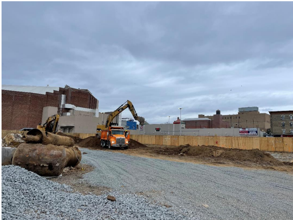
Photo 2: View of contractor loading soil on lot 14, facing northwest.
