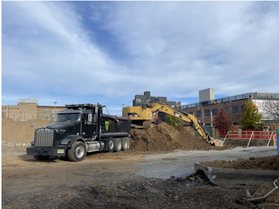
Photo 2: View of contractor loading soil in Lot 14, facing northeast.
