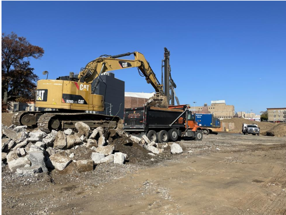
Photo 2: View of contractor loading C&D in Lot 14, facing west-southwest.
